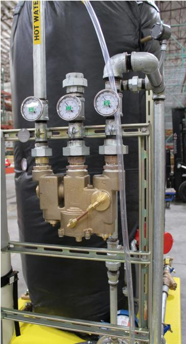
TEMPERING WATER for Emergency Equipment requires more functionality than is built into most mixing valves.
